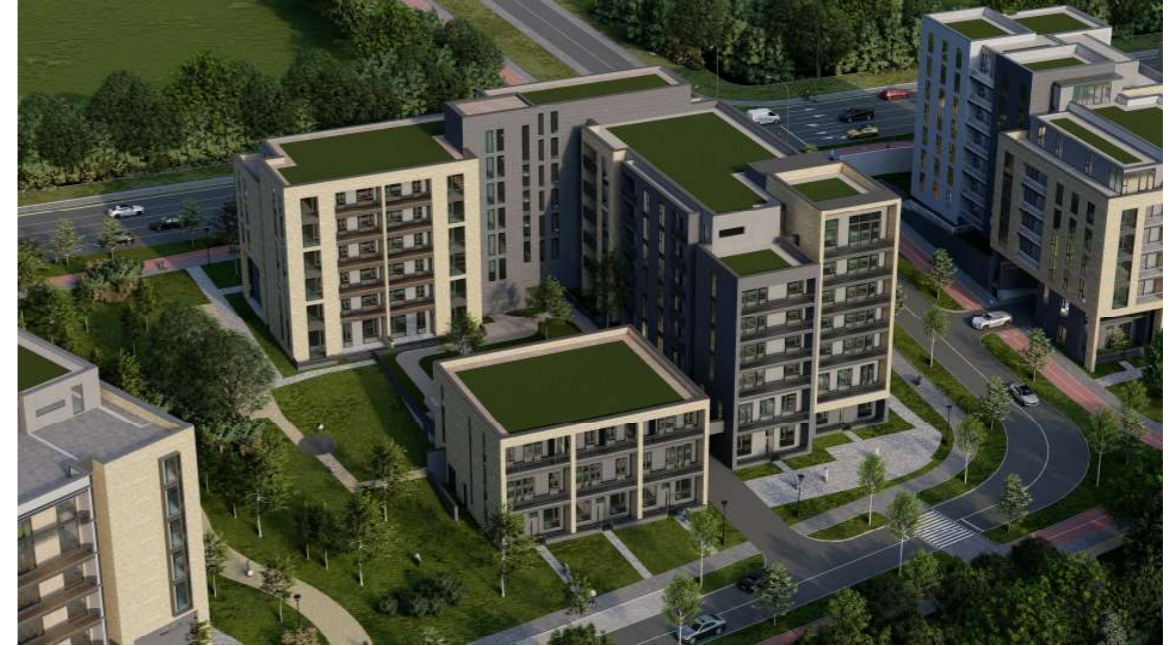
Block 5 aerial view
